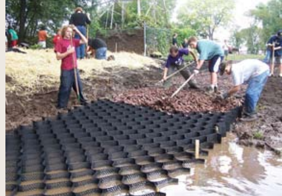
Scouts put into place the reinforcing GeoWeb
