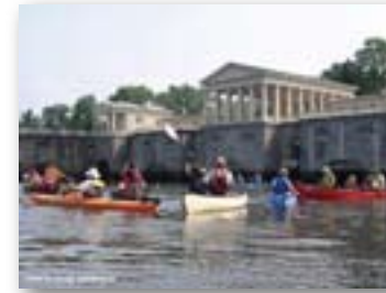
The Fairmount Waterworks from the tidal section of the Schuylkill River. Photo by Dennis DeFrancesco.
